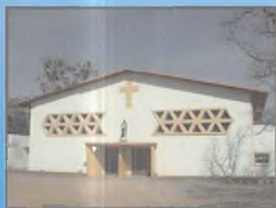
Shambyu - St. Joseph's Parish
