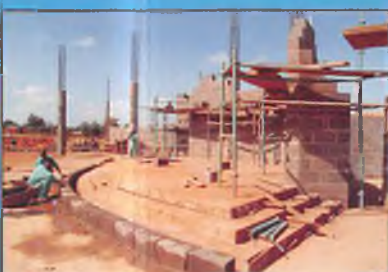
Lilongwe - Church under construction
