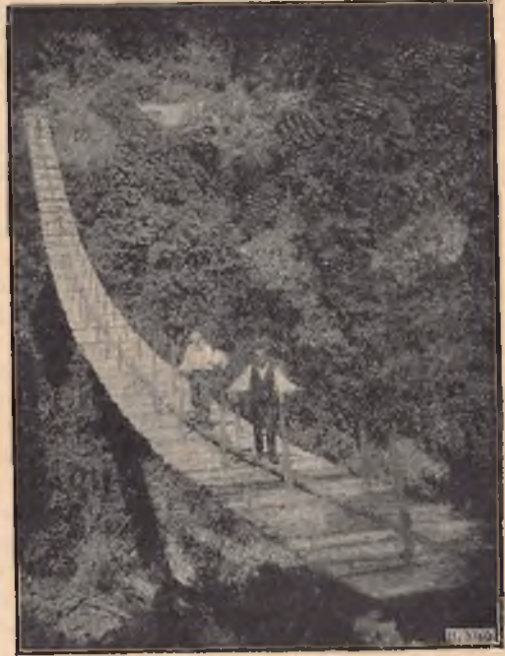
Mendez, Ecuador. — 'Suspension' Bridge built by the Salesians. 258 ft. long; 144 ft. high; 12 ft. wide.
